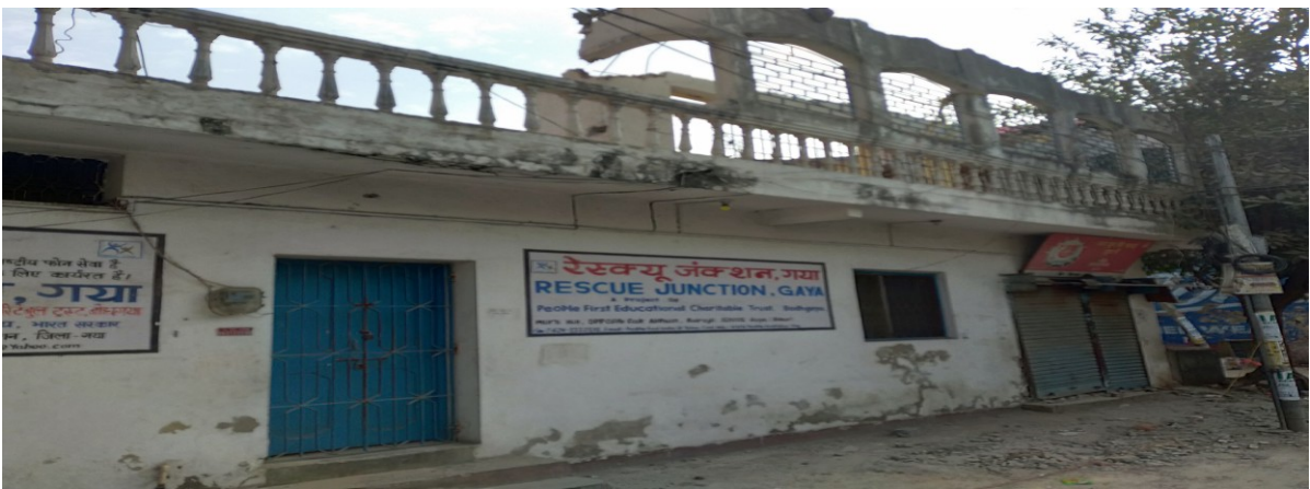
Old Rescue Junction Gaya during demolition
