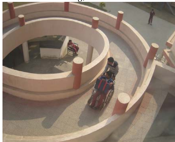
Ramp to Second floor
