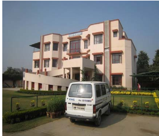
KWS Building, Garden and Van
