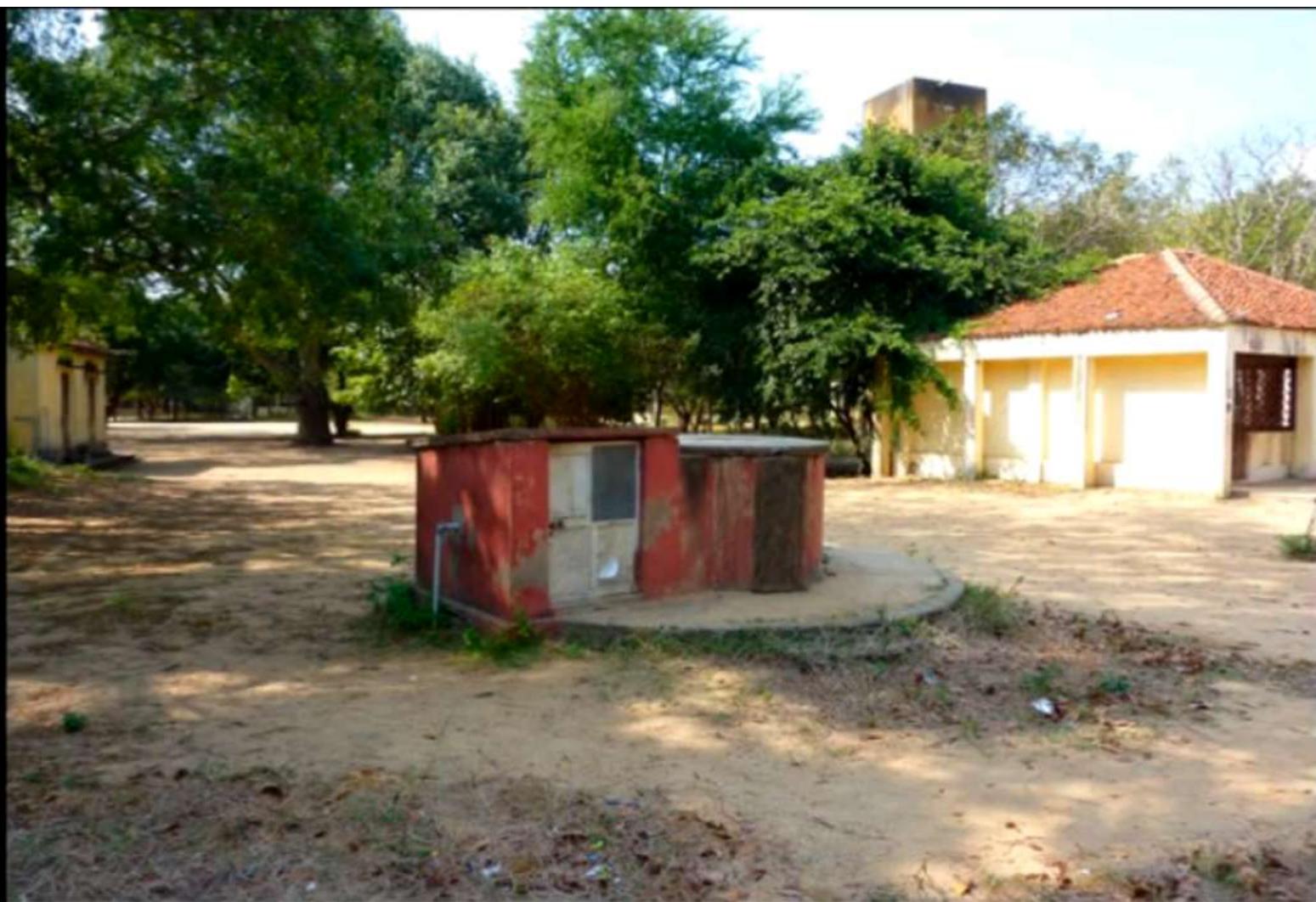
Outside the High School Toilets - Pump with Water Tower beyond.
