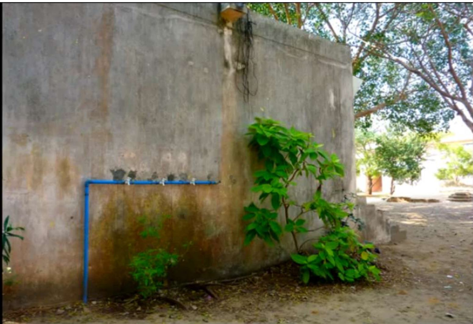
[OLD STYLE TAPS]: Inadequate number of taps are also mounted unproductively high. Children make a mess while washing their bowls, and have dirty legs from the spatter of food and water. More water is wasted in clean-up.
