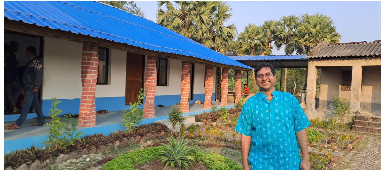
Newly renovated govt. school
