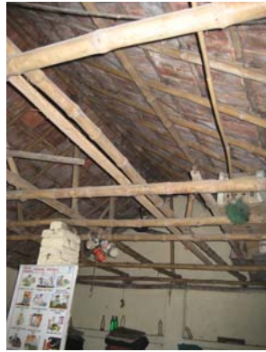
The roof of the night shelter.
