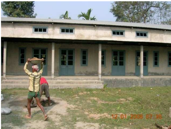
Class rooms construction (funding for this construction is from university)
