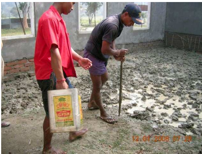
Work on Floor in Activity room
