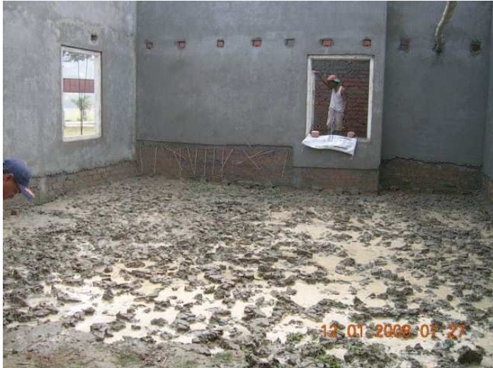
Ongoing work in Activity room
