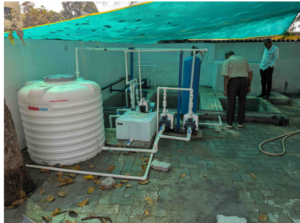
Image 2: Swimming pool for physical therapy. Image 3: Swimming pool water filtration system
