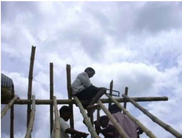
Construction at Thulir
