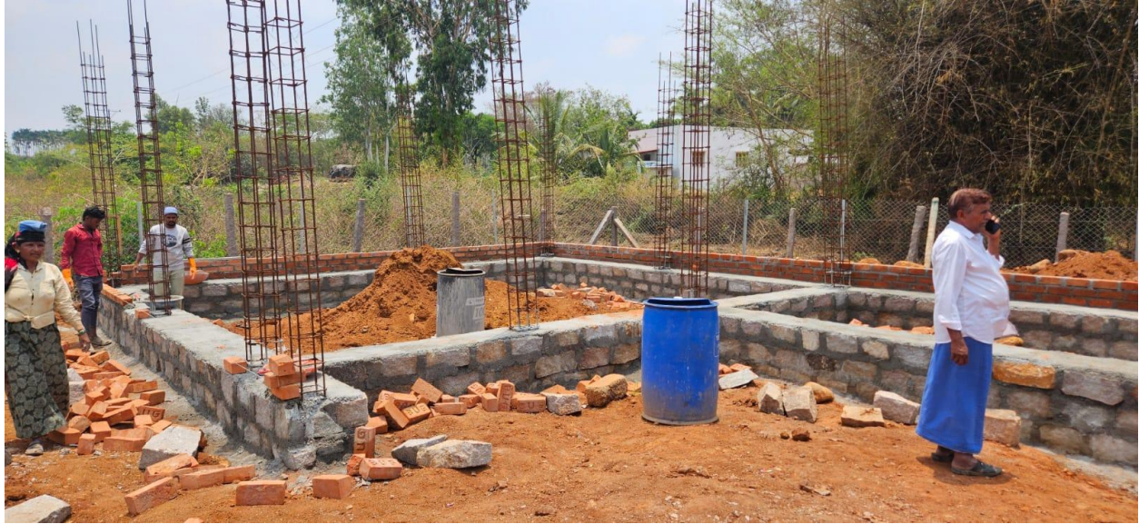
Images 1 & 2: New Building Construction (Next to Shivaganga Project Office)
