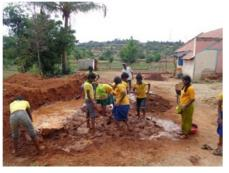
the material is local and all the children and teachers are pitching in to make this building happen. While we are doing the work we also experiment with various stabilisers and then test the bricks for compressive and tensile stress. The math involved is very challenging for the 7<sup>th</sup> and 8<sup>th</sup> graders, while the lower classes learn about the kind of soil needed to
