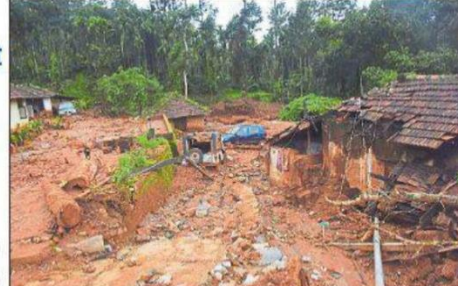
The damaged homes and snapped power lines, following landslides, have torn many lives asunder at Malemane near KotticHERA in Mudigere taluk of Chikmagalur district.
