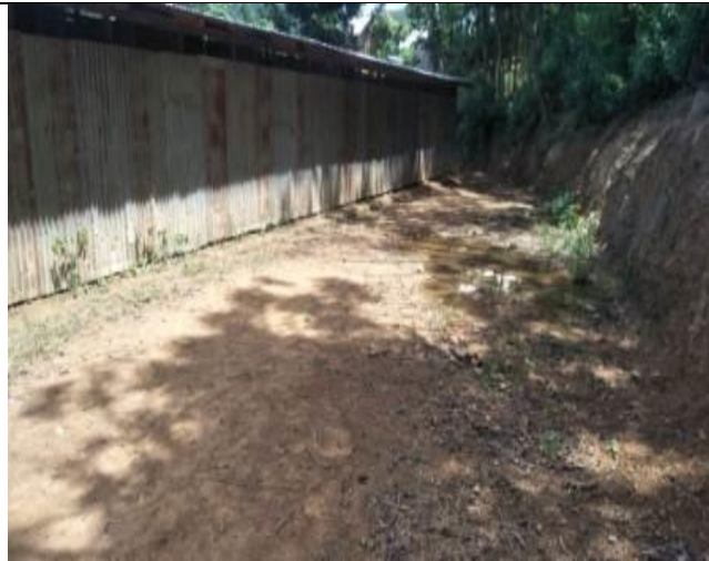
Wall conditions of 1 st school house made from iron sheet
