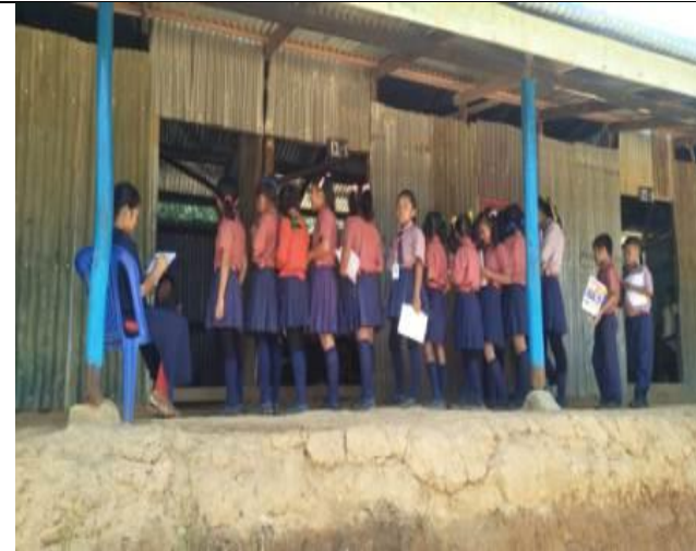
Plinth area of the school
