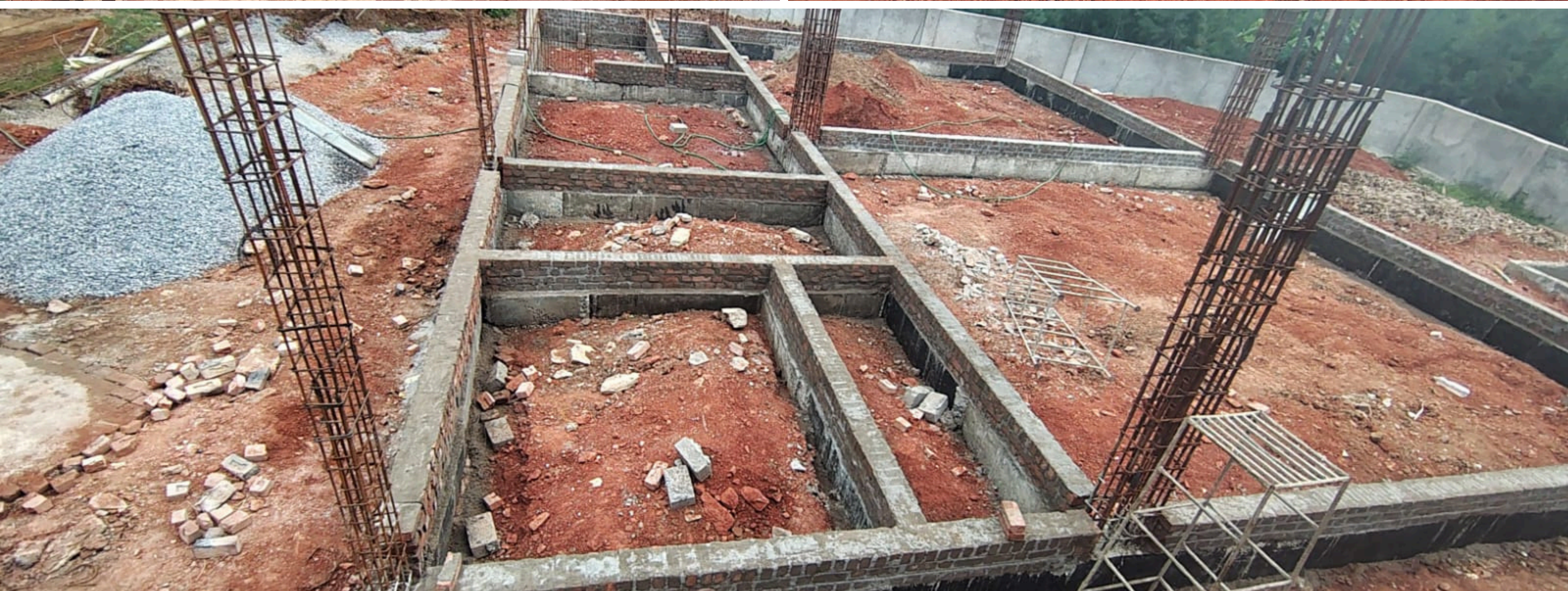
Foundation Construction & Ground Beam Work
