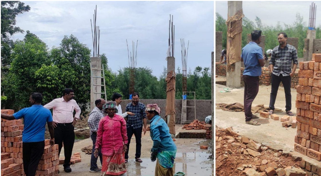
Brick masonry and structural frame under progress site visits by the Srujanavani and partner team
