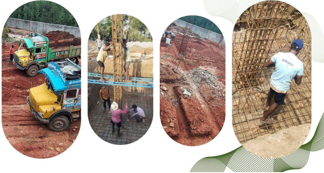
Soil excavation, footing and column foundation work
