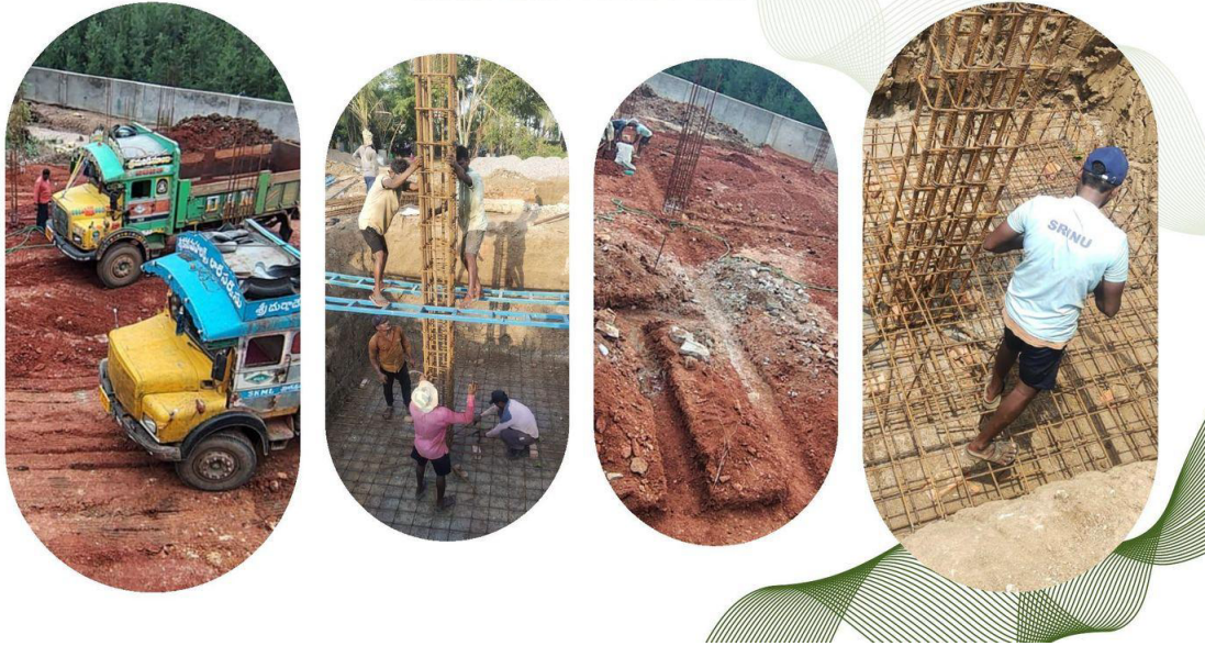
Soil excavation, footing and column foundation work
