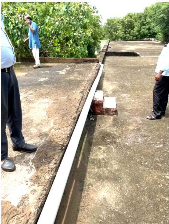
[clockwise from top] 1 &2. Inspecting the piped installed in the rooftop to feed rainwater into the water tank.
