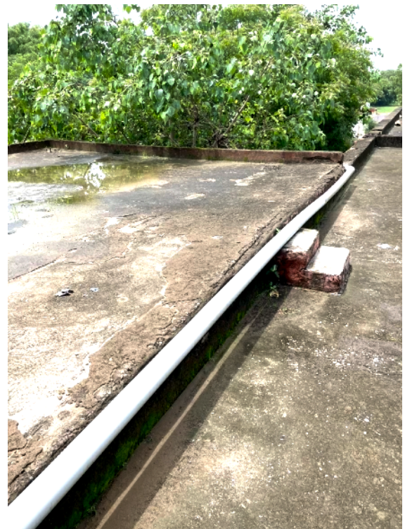
[clockwise from top] 1 &2. Inspecting the piped installed in the rooftop to feed rainwater into the water tank.
