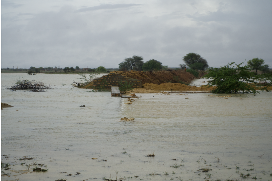
Water overflowing from a khadeen from the chaddar, protecting its embankment
