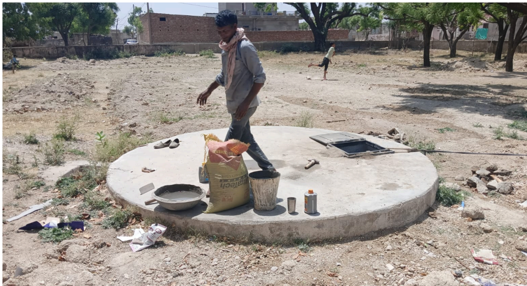
Repairing an existing tanka in a school in Jaipur
