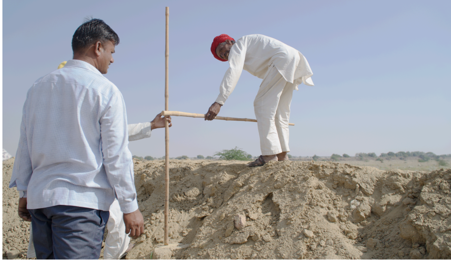
Making of an embankment in Jaisalmer
