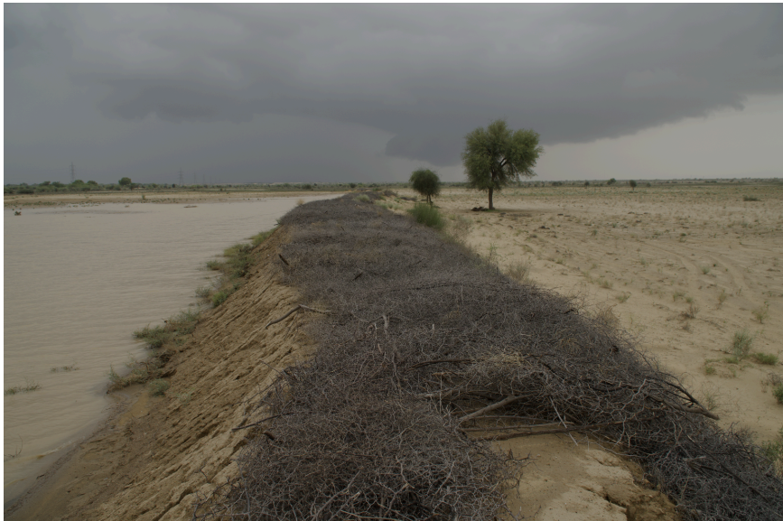
Chapai helps strengthen and protect the embankment in Jaisalmer
