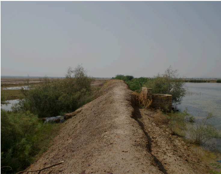
Different forms of Nalas were constructed using stone masonry and cement pipes to drain water from the khadeen
