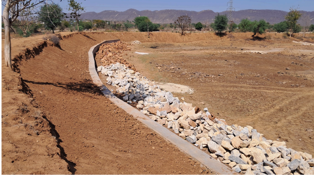
Making of a Johad, post excavation in Alwar
