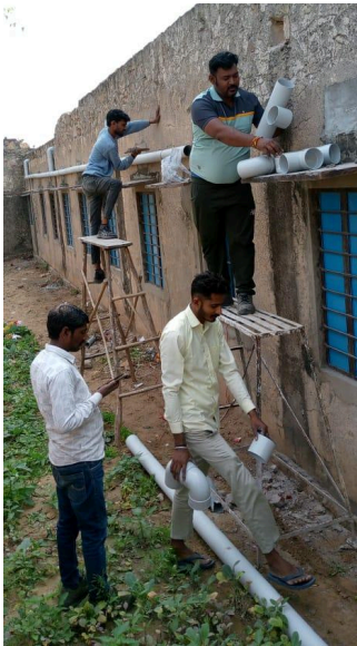
Pipes from the terraces were connected to the tanks to harvest rainwater
