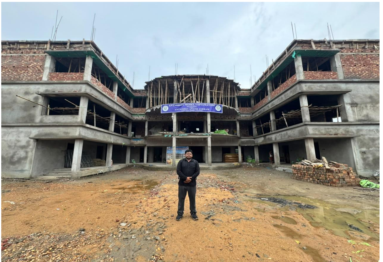
Standing in front of the newly constructed Antyodoy Model Vidyamandir High School
