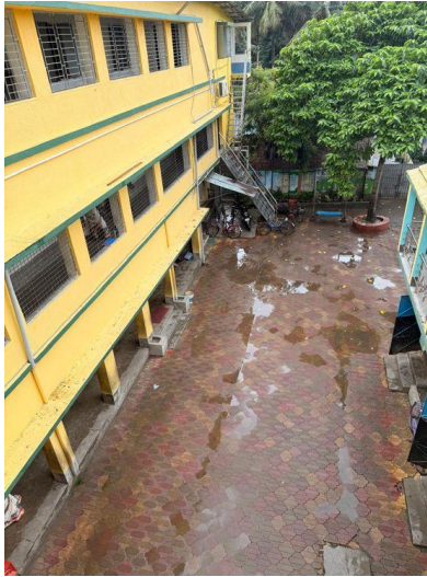
View from second floor
