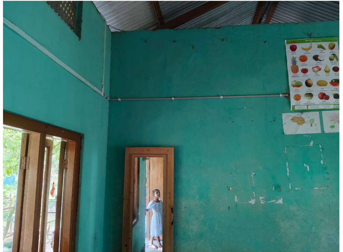
Classroom Building: Peeling and deteriorating paint on interior walls | Exterior walls show visible marks and stains
