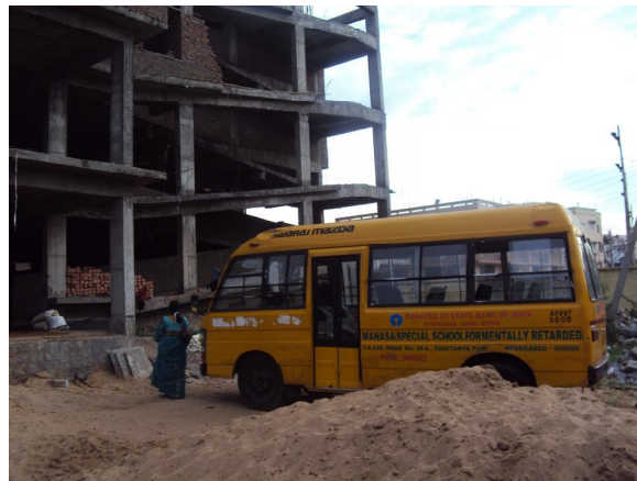
Pictures of the construction site clicked on July 1st
