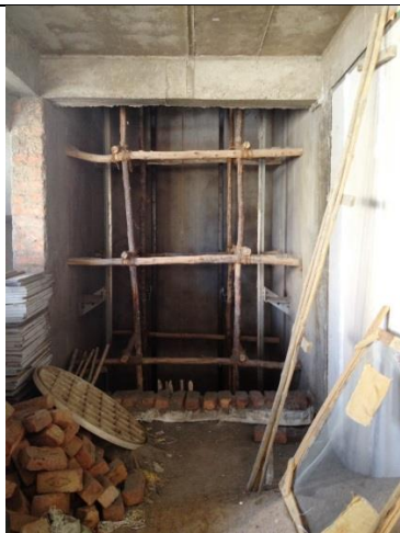
Elevator Shaft – Under Construction
