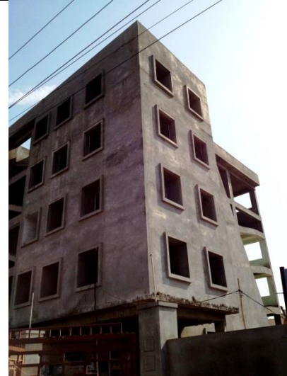
Overall 4 Floor Building
