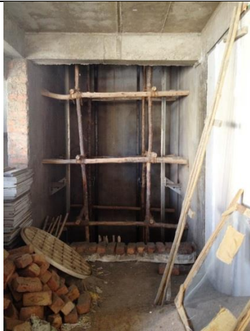
Elevator Shaft – Under Construction
