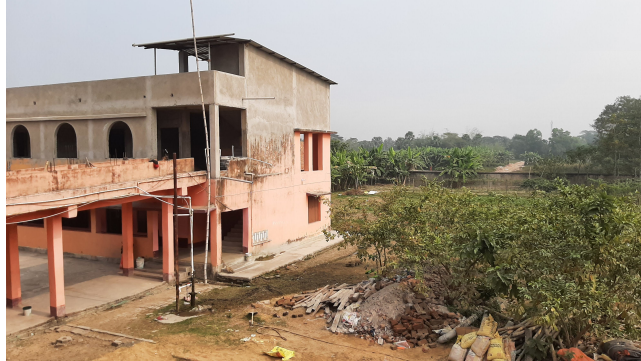
FIGURE 1. Construction of new floors at Tongtala Center
