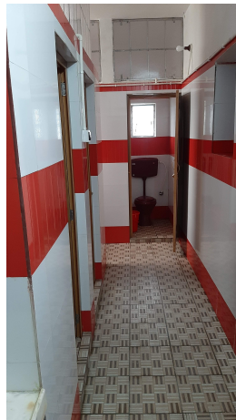
FIGURE 10. Newly constructed toilet block
