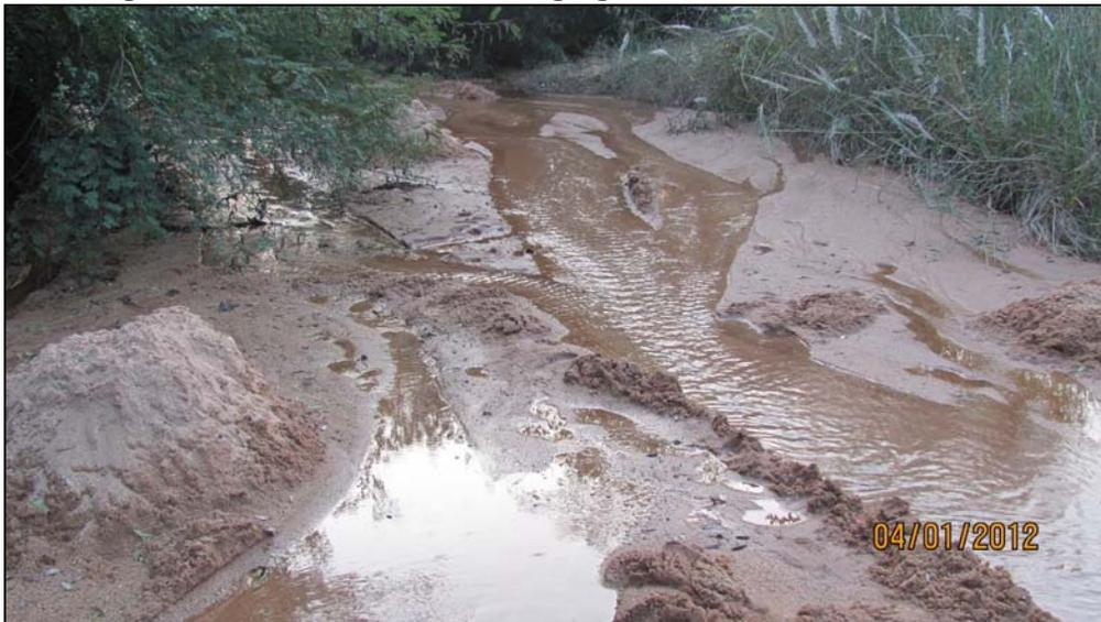
Photo- 7: One of the check-dams heavily silted
